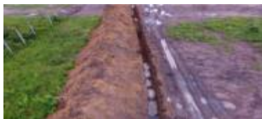
Figure 31: Combination of barricade and ditch to protect Águas Verdes. Sparta Solutions report.
