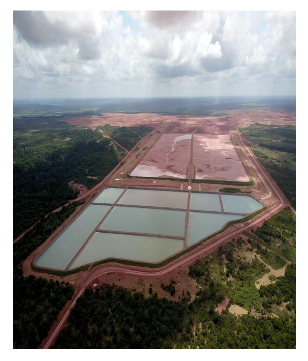
The TDA of Mineração Paragominas S.A. consists of four disposal quadrants (TDA-A, TDA-B, TDA-C, and TDA-D) delimited by internal and peripheral dikes and is responsible for the temporary drying of the tailings generated from the beneficiation of bauxite ore.
