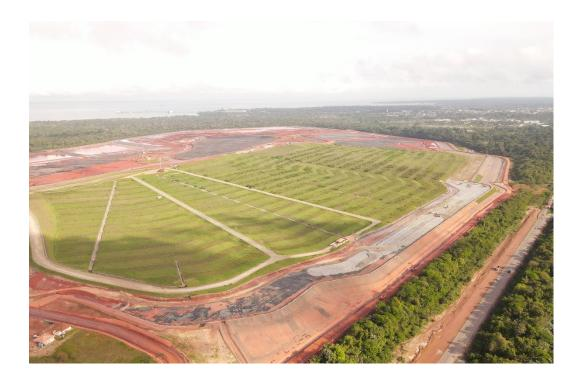
The closure is divided in 11 strips of rehabilitation. The strips 2, 3 and 4 have been rehabilitated, and represent approximately 60 ha. The design considers cap and store the filtered residue with cover systems consisting of HDPE geomembrane to lining the stored residue, covered by a densified soil, and revegetation of the surface.
